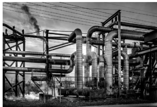
Steel Mill Steam Pipes
